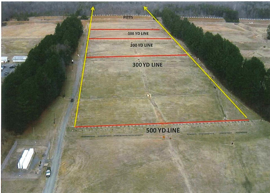
Overhead view of Range 2
