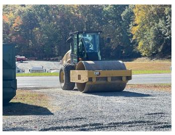
**Public Works** completed a QSC work order to roll the parking lot and use millings to build the area level around the shotgun trailer. This leveling allows us to (now) easily back trailers delivering pallets of clays for the club.
