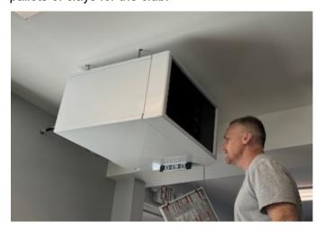
A new propane heater was recently installed in the clubhouse to replace the 23yr old unit. The old unit was noisy and held up by drywall screws (yes, drywall screws). We had certified gas installers suggest a new unit and then conduct a proper sighting, fitting and installation. The new unit is more efficient and designed to offer years of quality service. This replacement represents a \$4,700 investment that was paid for using match proceeds.
